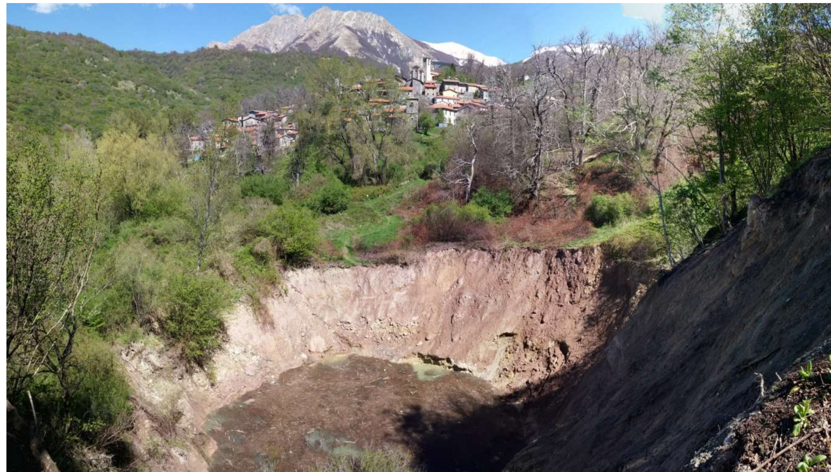
Sinkhole, collasso Sassalbo, 2017
